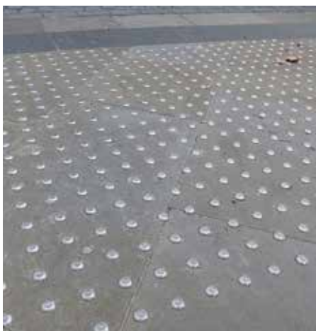
Raised metal tactile studs at crossing points, set in natural stone
