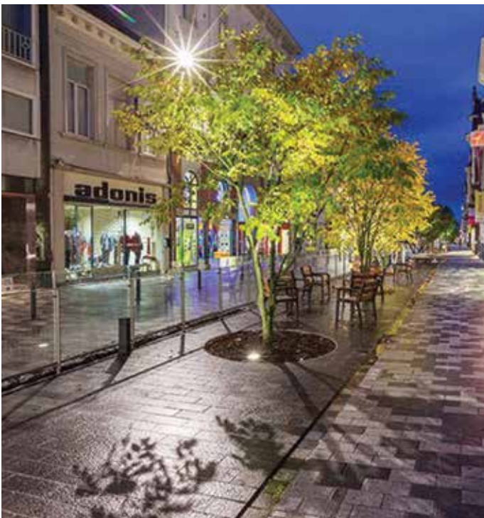
Below: Public Realm project at Stationsstraat, Sint-Niklaas, Belgium
